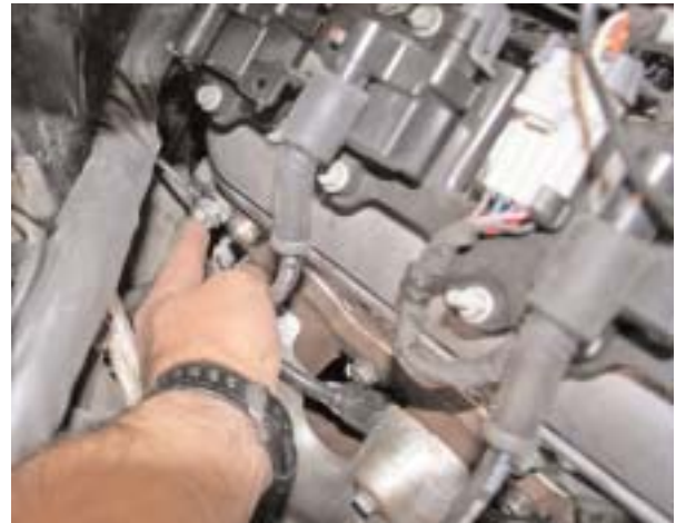
The computer engine harness is grounded to the back of the passenger side head. All grounds must be clean for a good contact. Battery to engine, engine to frame, engine to body are all needed to insure proper operation.
